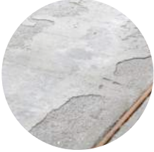
Spalled Concrete
